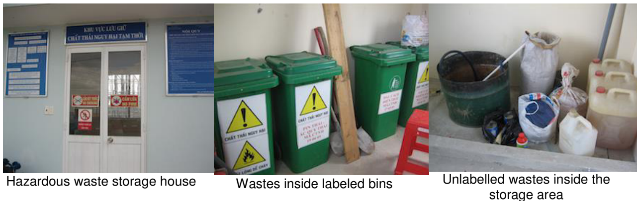
Photo 6: Hazardous Waste Storage Area
