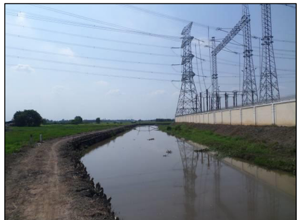
Irrigation canal at southern area of S/S
