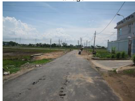
Access road to substation next to staffhouse
