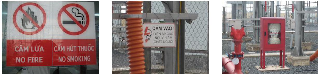
Photo 8: Safety warning signs and fire control measures at the substation
