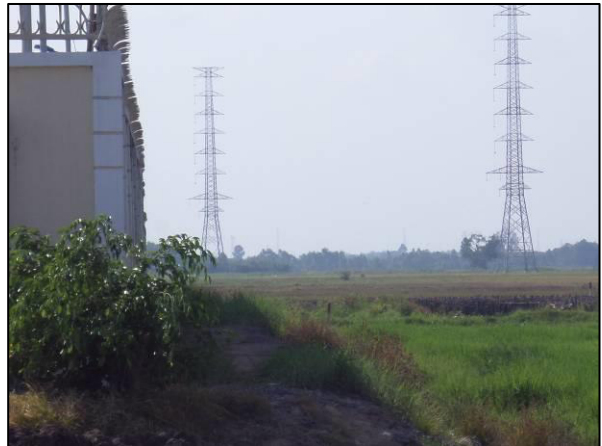
At the northern section of the substation
