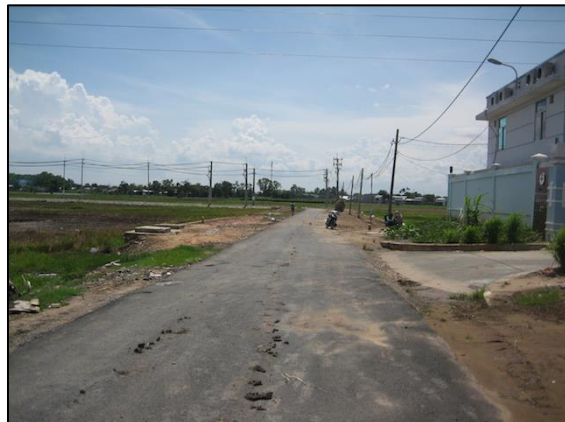
Access road to substation
