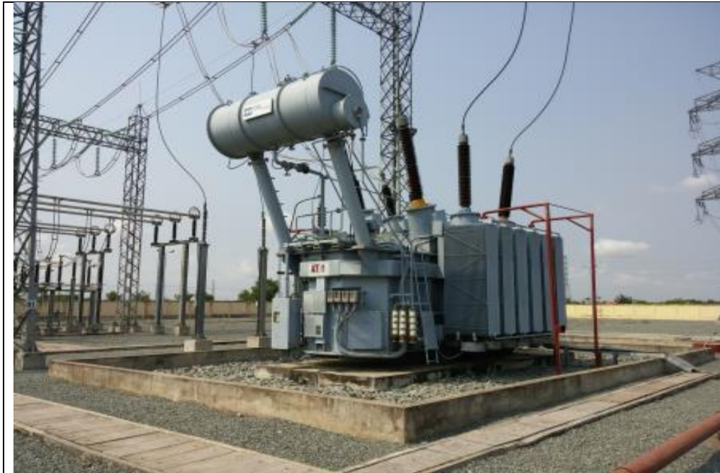
Fig 4b: Existing Transformer
