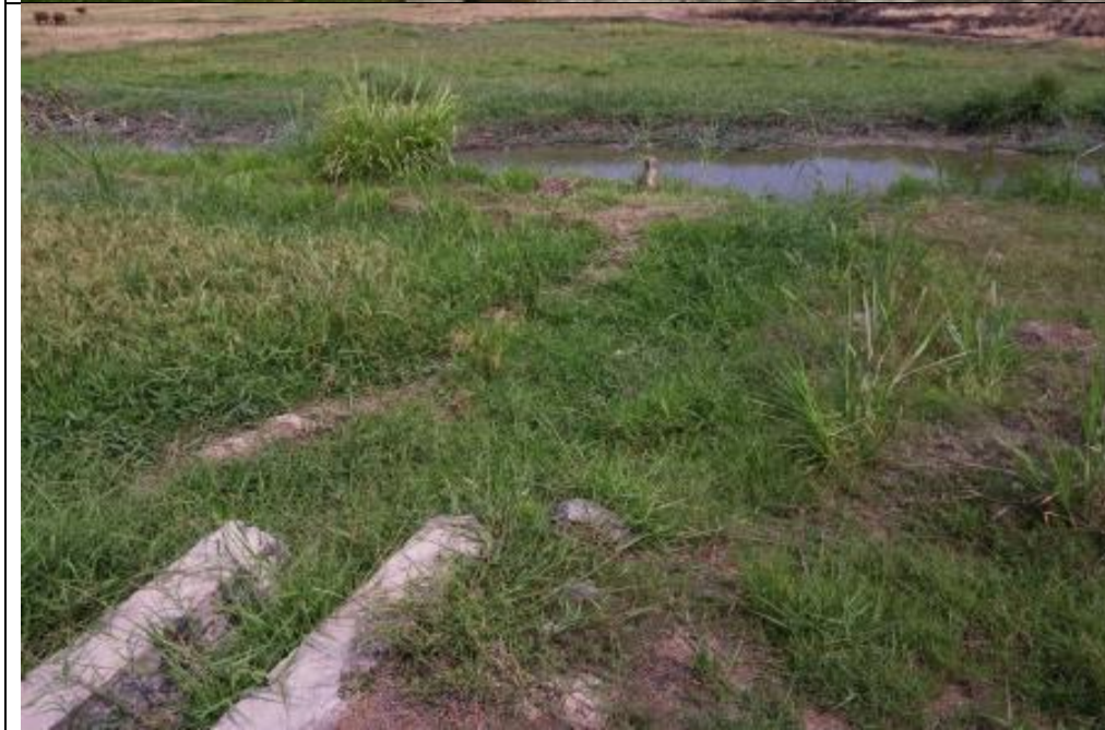
Fig 4e: Wastewater discharge to irrigation canal
