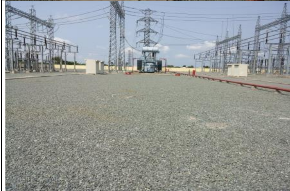
Fig 4c: Location for newtransformer
