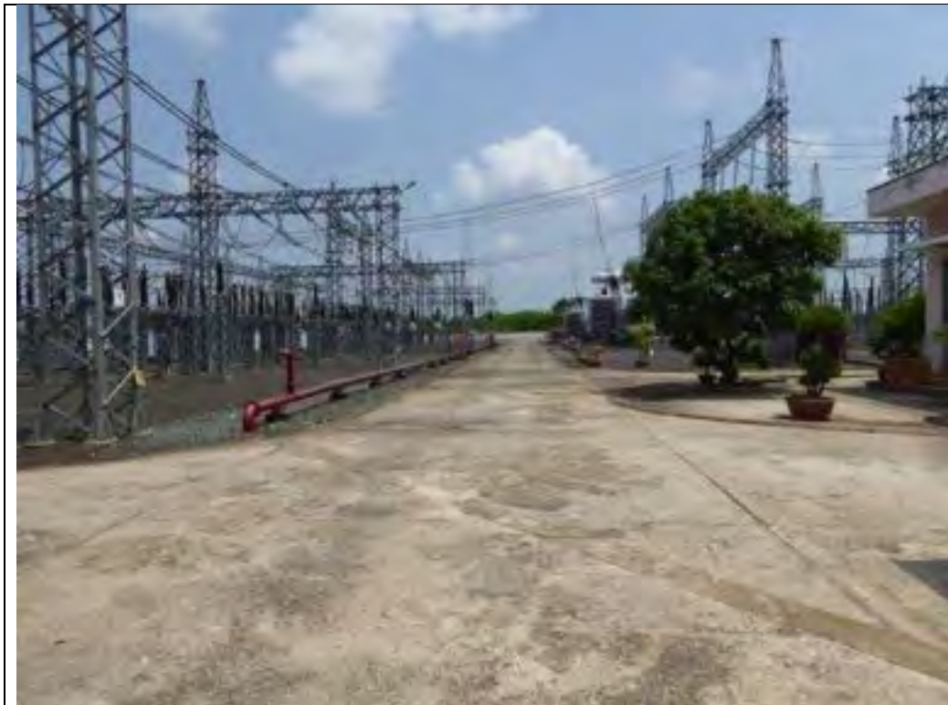
Fig. 4a: 220 kV Binh Long substation.
