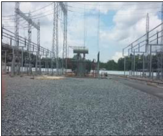
Current 250 MVA transformer
