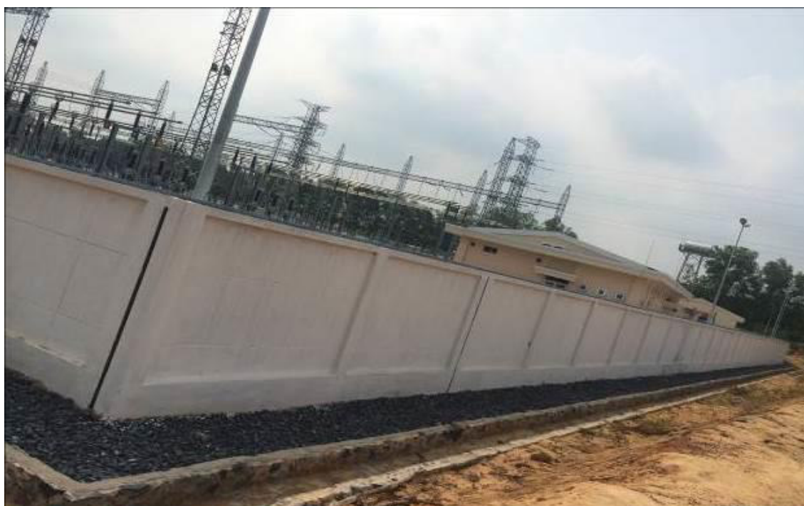
The drainage surrounding the substation
