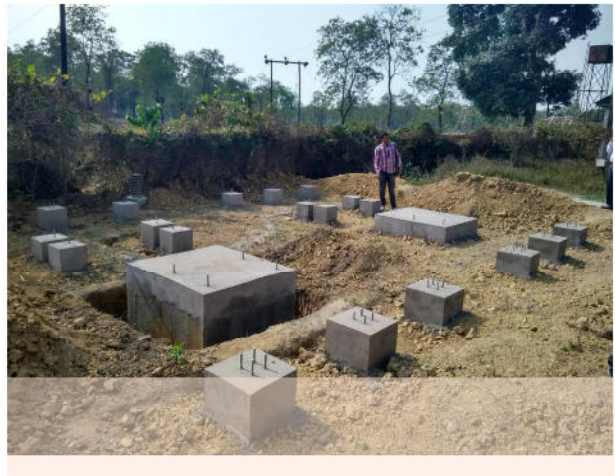
Photo 2: Foundation construction at Hazelbank S/S
