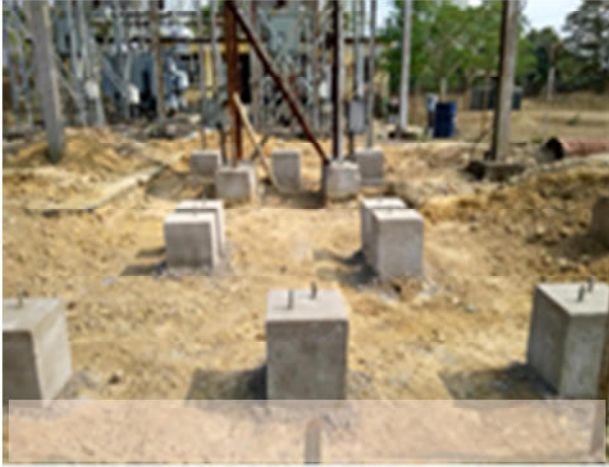
Photo 1: Foundation construction at Chabua S/S
