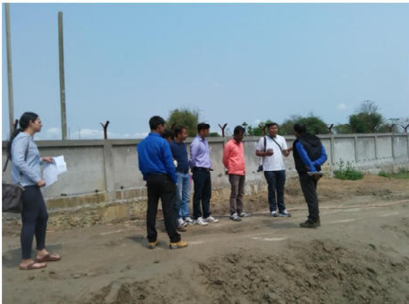
Photo 3: Interacting with the Contractor at Bedeti sub-station site
