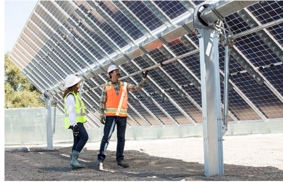
Figure 23: PV tracking system and inverters (Single-axis trackers follow the sun east-to-west on a single point)
