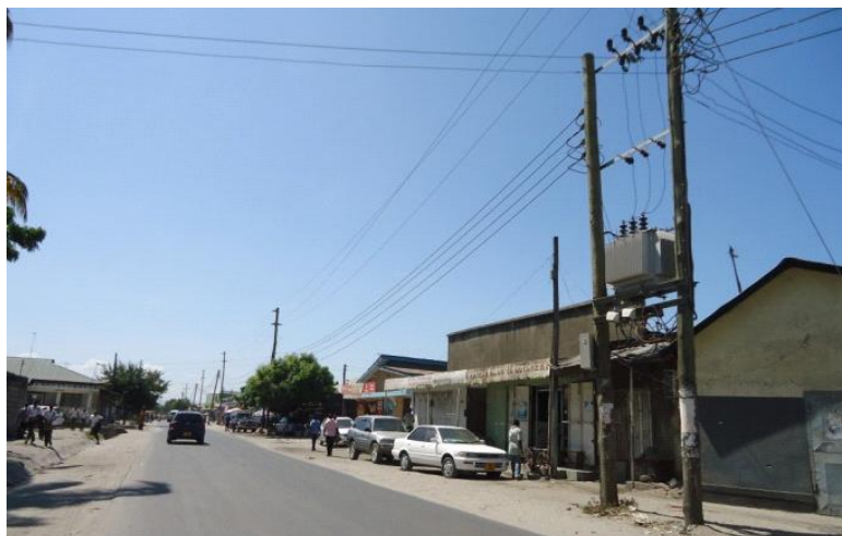
Figure 5.3: Power Transmission line just near the Makanya Subproject
