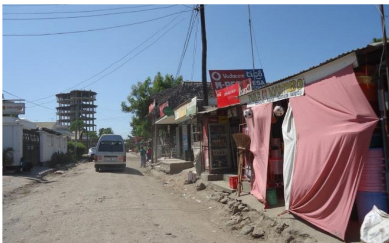
Figure 5.2: Shops very close to the Simu 2000 subproject
