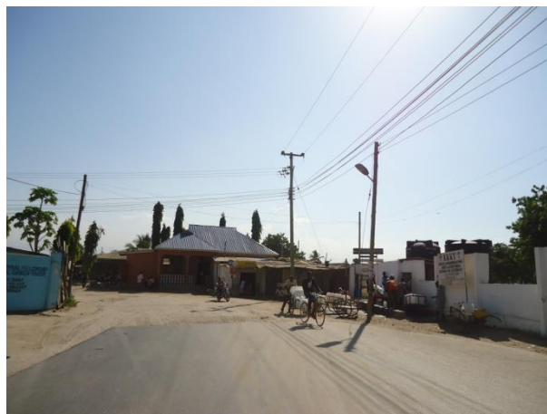
Figure 6.3: Power Transmission line Along Mchicha Subproject
