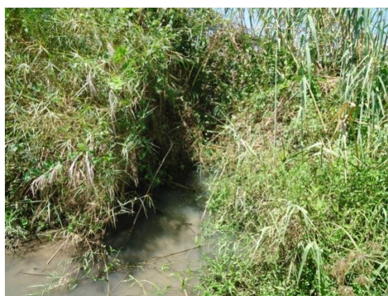
Figure 6.4: Kizinga River where Tuangoma Bridge Subproject shall be implemented
