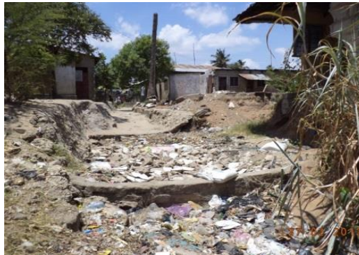
(Field work, PROCESL/COWI, 2014)
