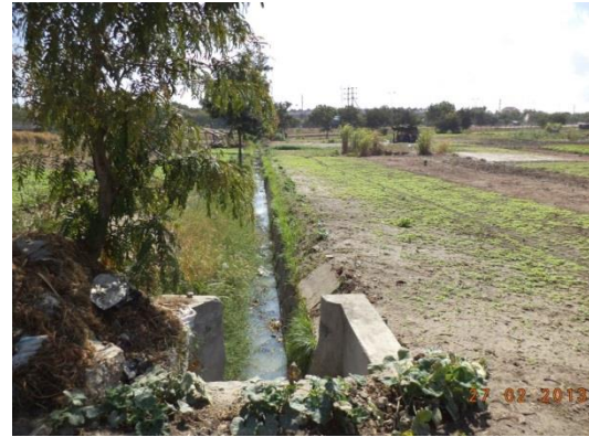
PHOTO 2 TEMEKE UNDERGROUND DRAIN
