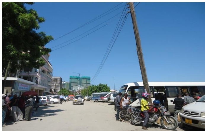
Figure 6.3: Power Transmission line just near the Kiungani Subproject
