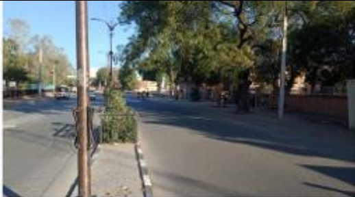
Railway hospital to JDA circle
