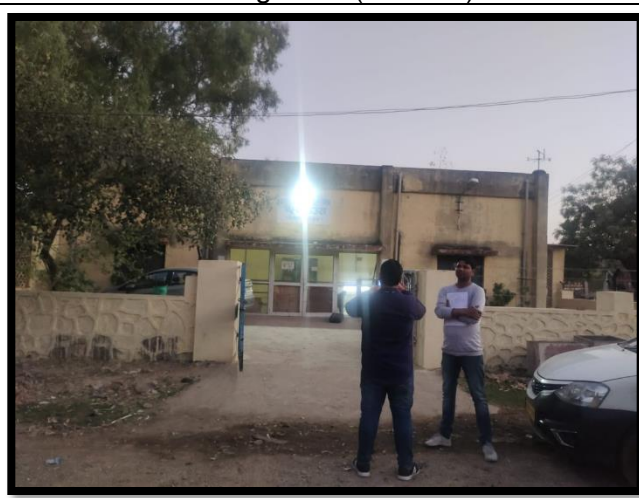
Existing OHSR at Vikas Nagar
