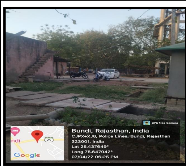
Existing CWR at PHED campus, Nainwa road, Bundi
