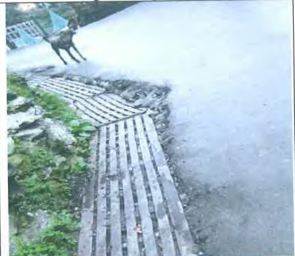
Blocked & uneven drains beside the road to Ridge to Chalet Day School
