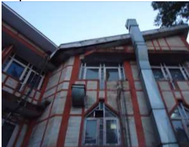
Figure 11: Exhaust Duct from Pantry & Kitchen
