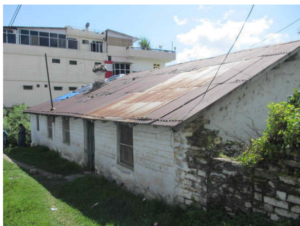
1. Existing Tehsil Quarters
