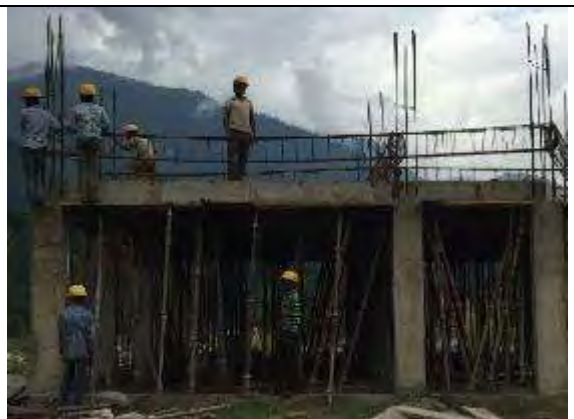
Safety measures neglected – no fire extinguisher & no safety belt being used
