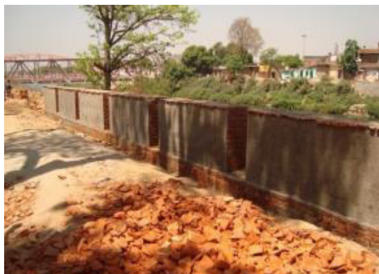
View of Construction Work of Guard Wall in Progress at Upper Ganga Canal bank
