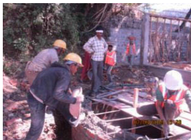
Concreting work for water storage tank
