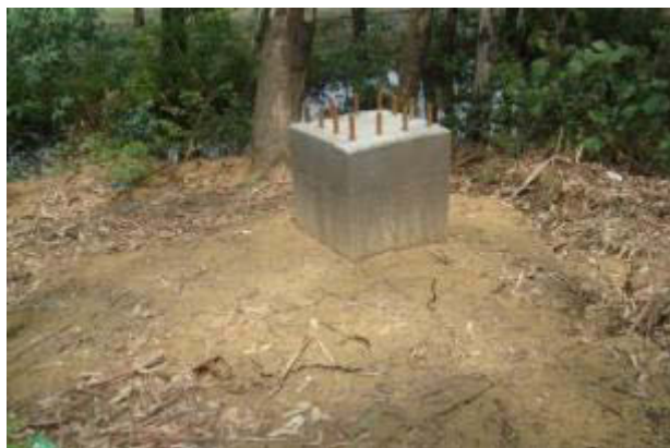
Work in Progress for Laying Foundation Type 1 for Signage at Jaspur ( Udham Singh Nagar Dist.)
