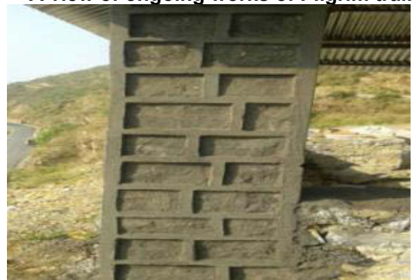
Pointing work at viewing shelter
