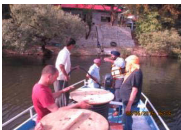
Installation of Aeration Discs and tubing
