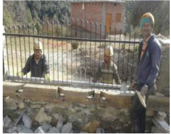
Ongoing railing work on Boundary Wall
