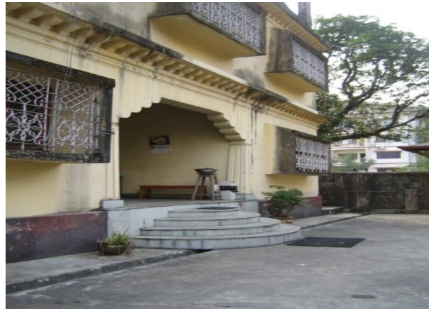
Affected structure, still occupied.
