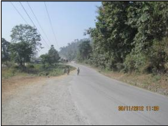
Photograph 2 2 nd Pole to 4 th Pole
