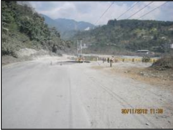
Photograph 1 Bridge (east end of Pasakha Access road)
