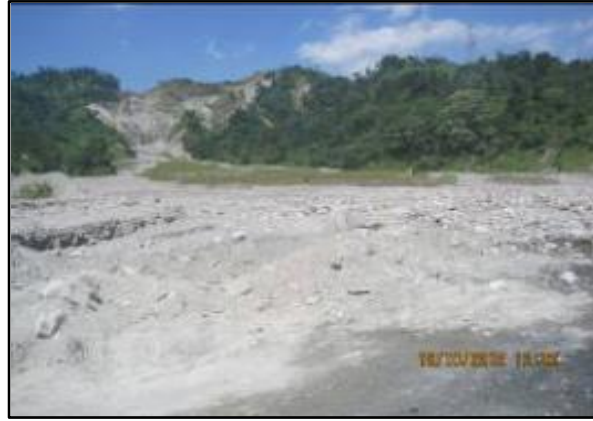
Photograph 4 Land slide area
