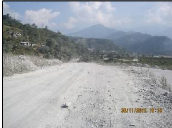
Photograph 5 Temporary road across land slide
