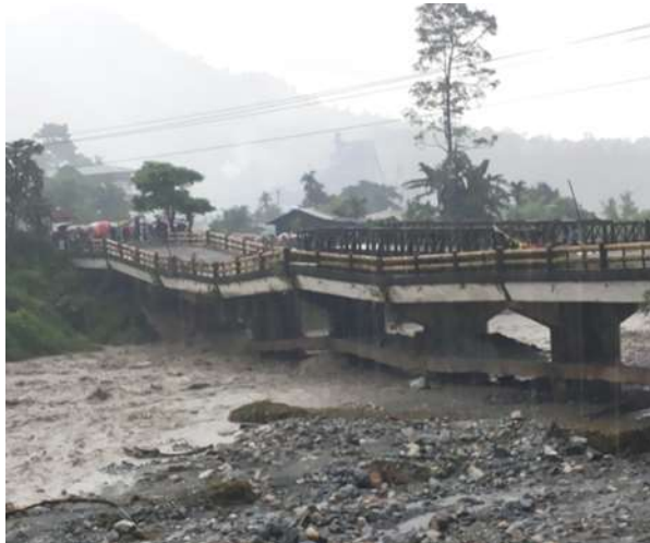
Picture 15: Bhalujhora bridge damaged by floods
