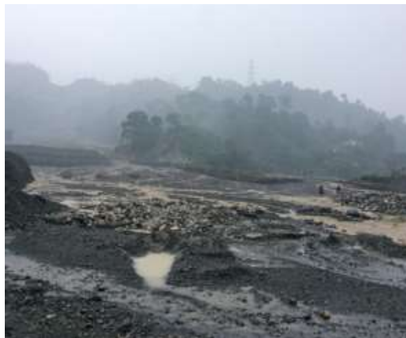
Picture 14: Siltation of work site due to flooding at Bhawanijhora
