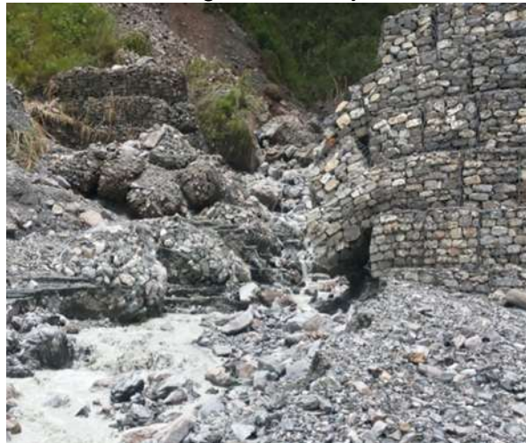
Picture 16: Gabion checkdams damaged by flash flood
