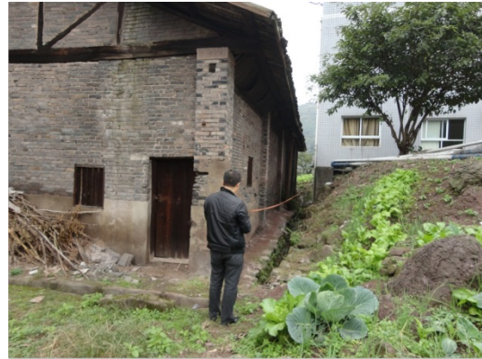
Right side of the warehouse
