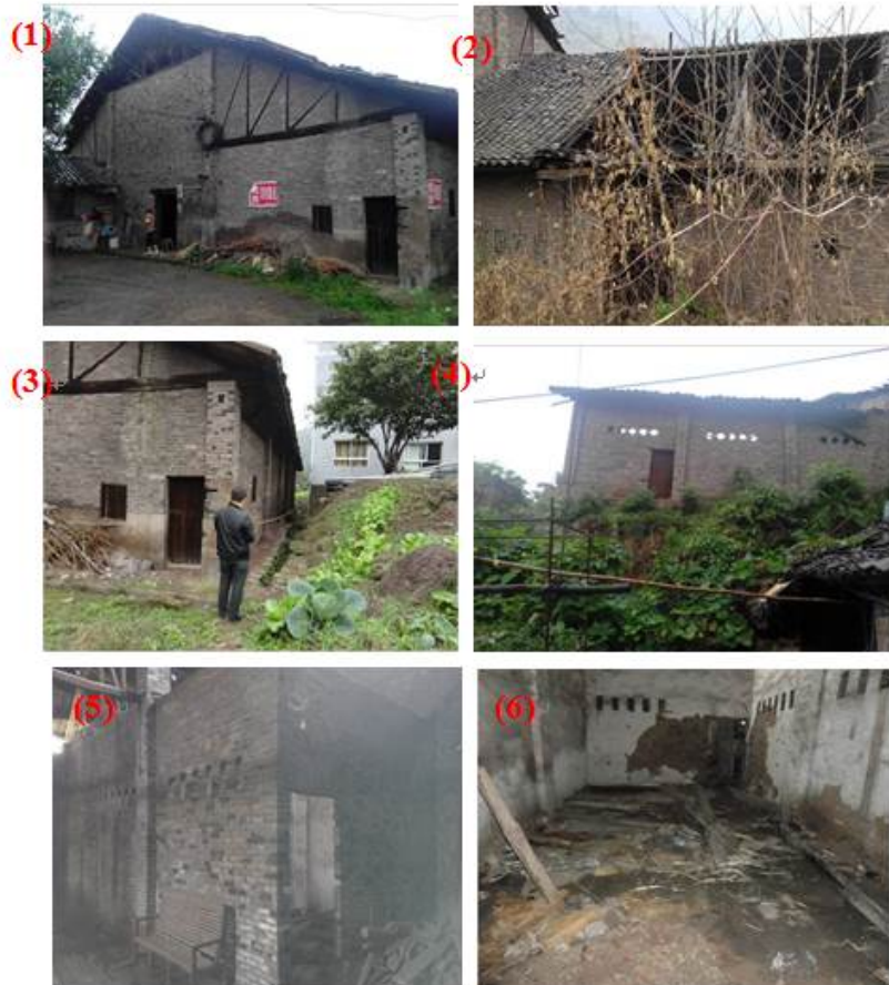
Figure 2 Status Quo of Ganshui Warehouse (1) Front side of warehouse; (2) Reverse side of warehouse; (3) Left side of warehouse; (4) Right side of warehouse; (5) Keeping room; (6) Pesticide storage room inside the warehouse.
