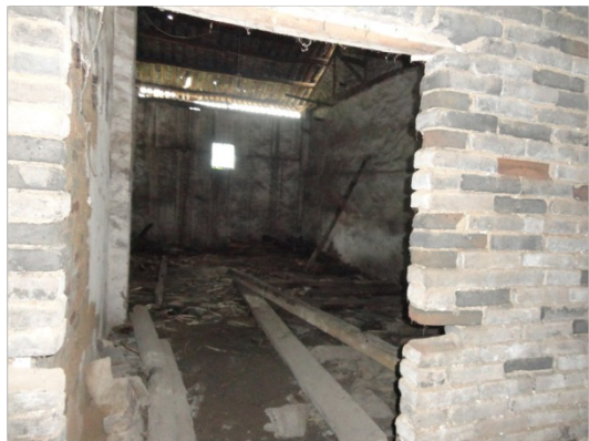
Inside of keeping room
