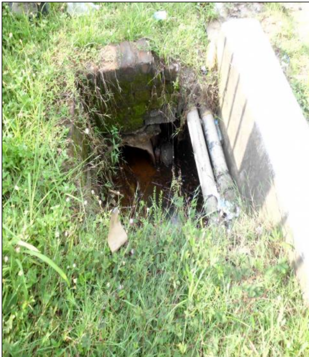
Figure 4: completely blocked lead away due to very poor maintenance
