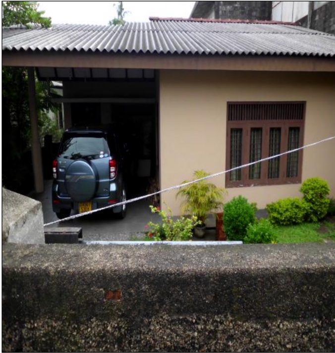
Figure 13: House constructed over the leadaway drain by completely closing the drain
