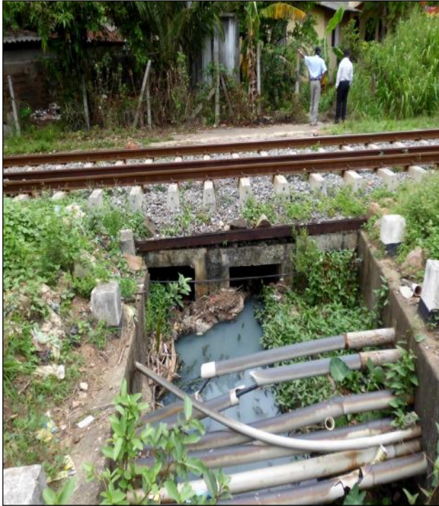
Figure 6 : Many utility lines blocking the water way path (Culvert 33/2)
