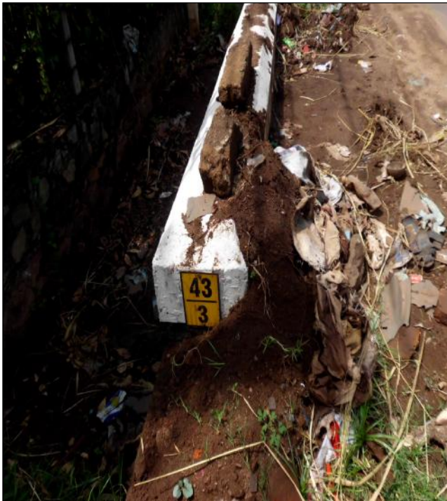
Figure 12: Completely blocked lead away
