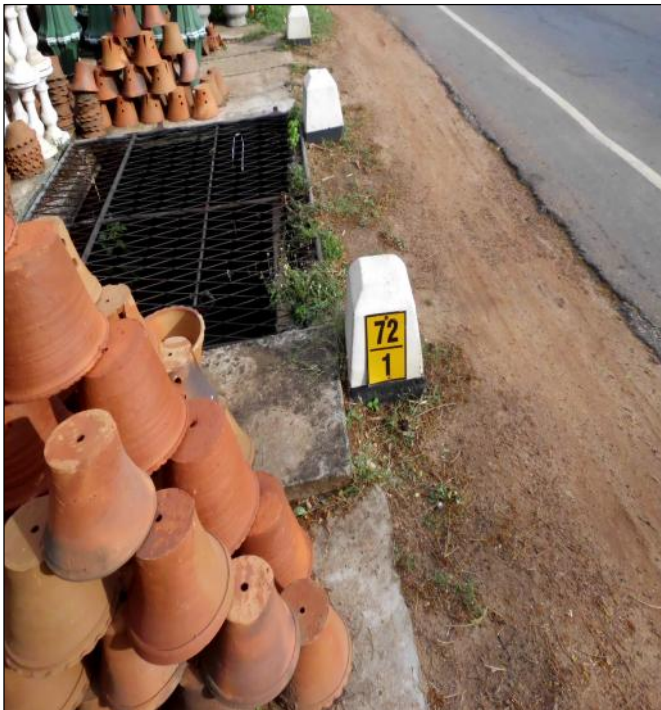
Figure 15 :Lead Away completely closed clay pot shop constructed on the waterway path
