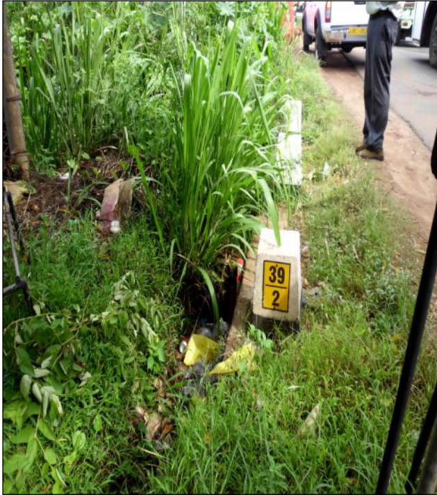
Figure 10: Neglected lead away drain
