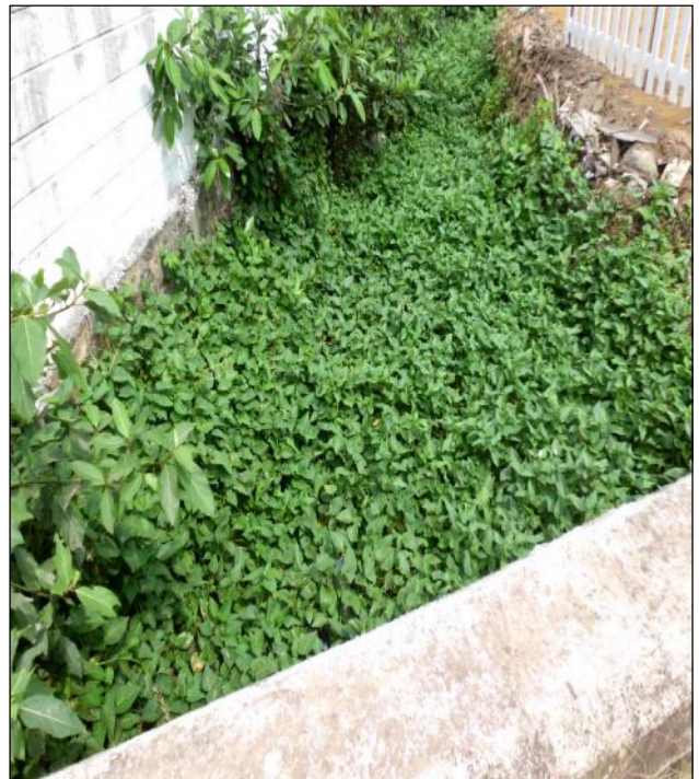
Figure 7: Totally blocked lead away with weeds and silt
