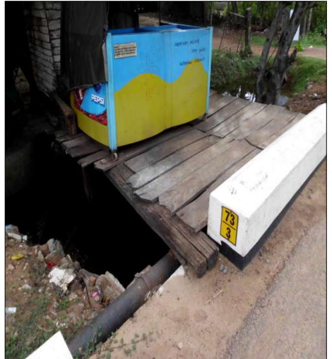
Figure 16 : Grocery shop on top of the leadaway path
