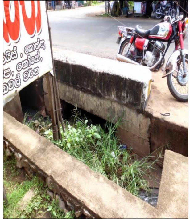
Figure 9 : Leadaway path is partially blocked
