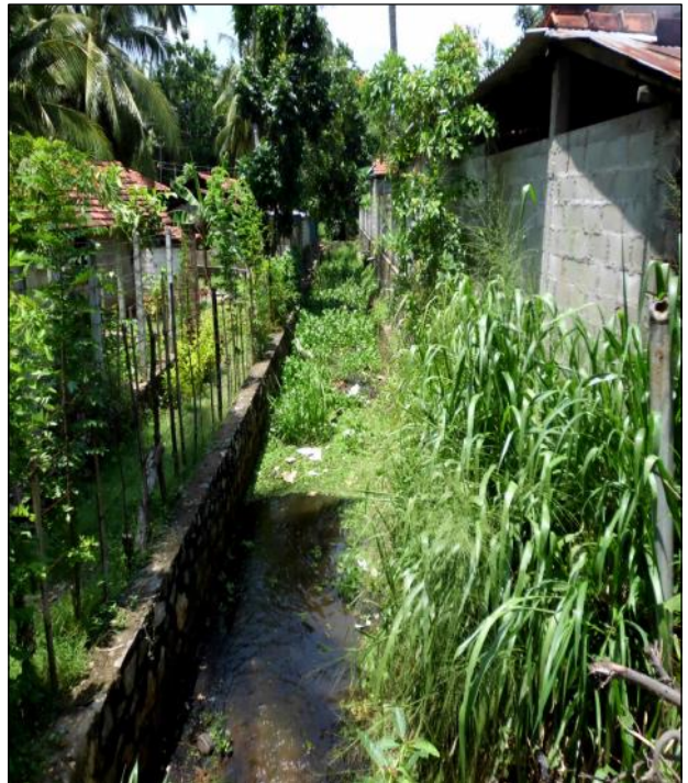
Figure 11: leadaway blocked by residents down stream
