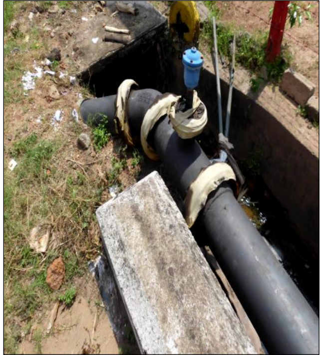
Figure 5: Main water line taken through the lead Away path (27/1)
