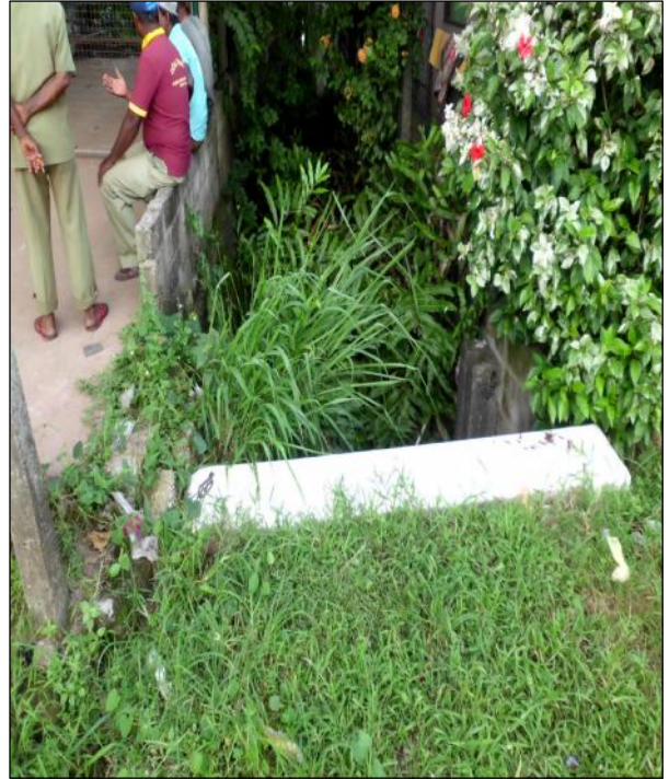
Figure 1: Lead away blocked downstream, heavy growth of weeds and siltation
