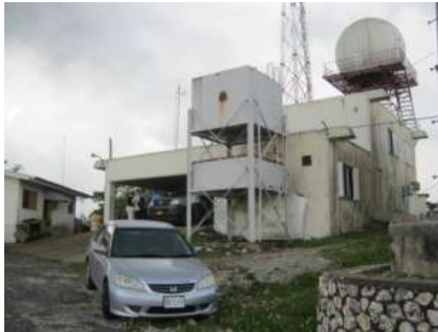
Plate 3.0 Current Radar installation at Cooper’s Hill
