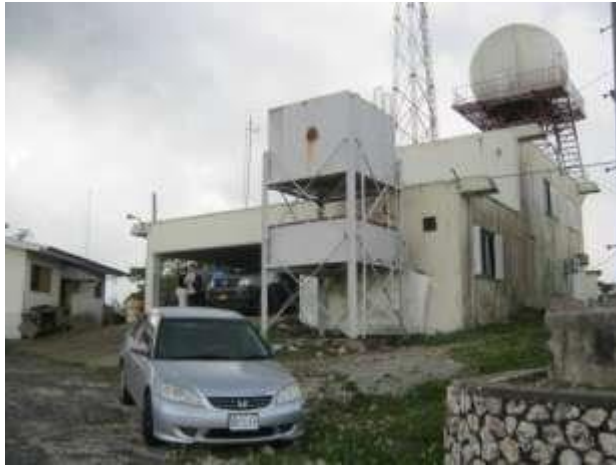
Plate 3.0 Current Radar installation at Cooper's Hill
