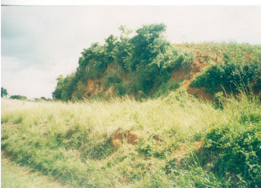
Plate 5: One of the abandoned borrow pits close to the road. The borrow pit is creating a visual impact to road users.
