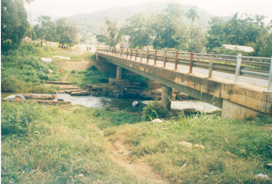
Plate 3: The Pangani River Bridge the river bed underneath is rocky (CH.13+500)
