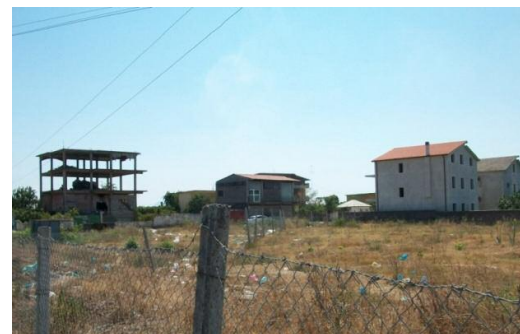
Figure 7 School site (view 2)
