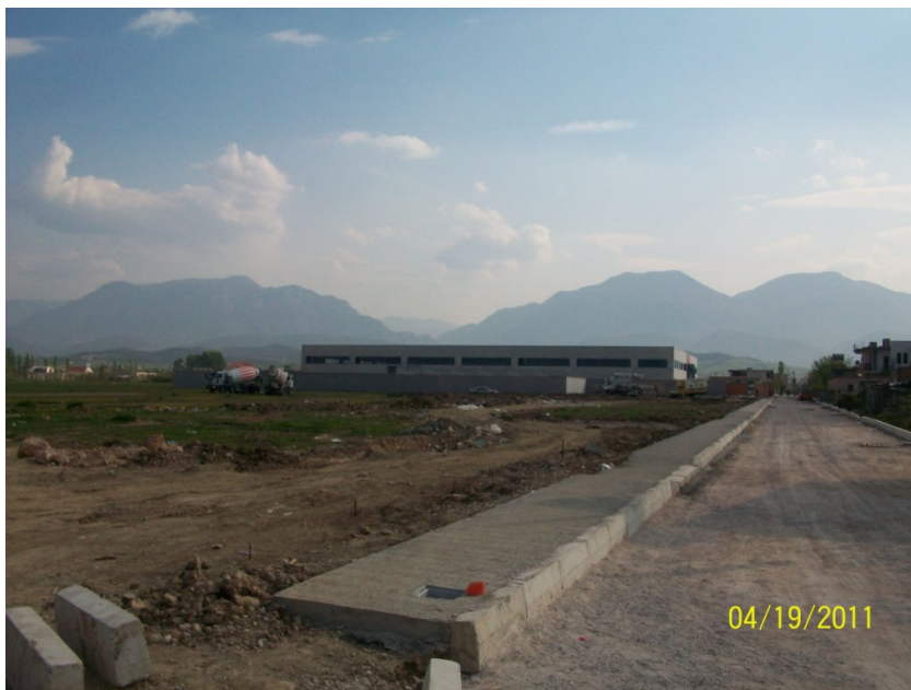
Figure 10 School site and road “Erzeni” under reconstruction.
