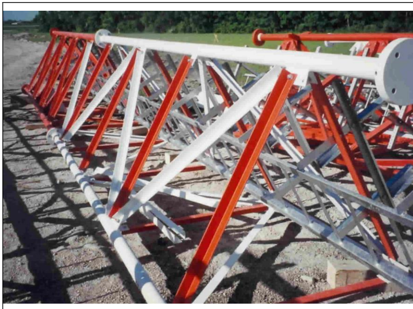
Photo 2: Stacking Tower Sagments at BTS Site Station
