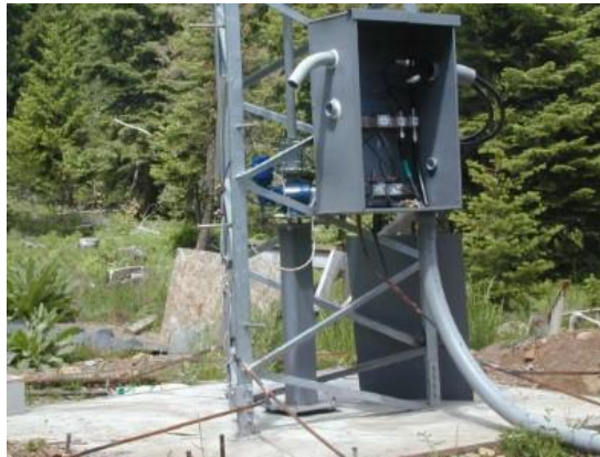
Figure 3.7 Lighting Protection Gear
