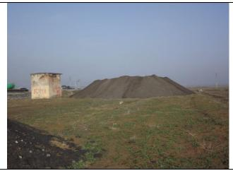
PK 138 Milled asphalt is stored on topsoil
