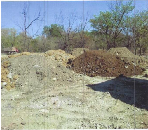
Private land plot (PK112) Mixing of topsoil and subsoil
