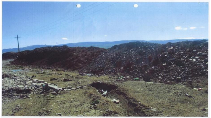
Section 3; PK132.80 Stored topsoil was mixed with gravel
