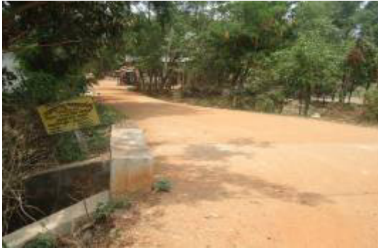
Start Point – ROW free from encroachment
