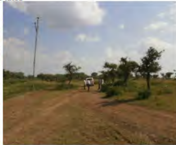
Ch-100m to Ch-200m HT line
