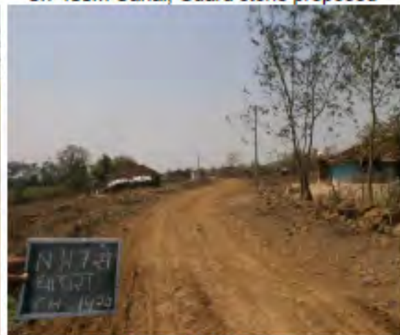
Ch-1400m Habitation area
