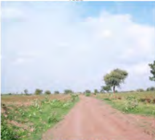
Ch-200m to Ch-300m
