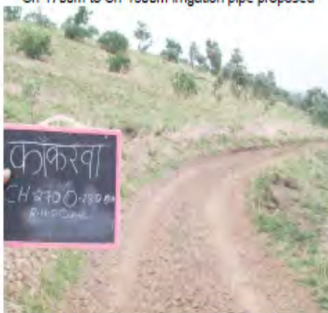
Ch-2700m to Ch-2800m Curve RHS
