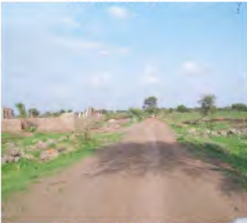
Ch-1000m to CH-1100m
