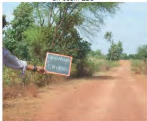
Ch-900m almost straight alignment
