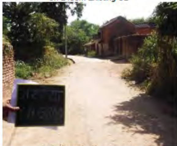
Ch-5800m Habitation area
