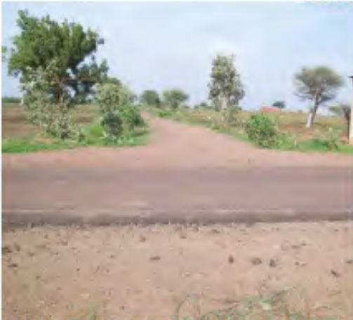
Ch-00m waiting room RHS at start point of the road
