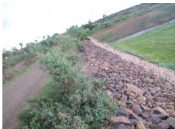
Pond at RHS, CH-4000-4100M Road Name: Dhatrawada to Kankarwa Block Name: Ratlam District Name: Ratlam
