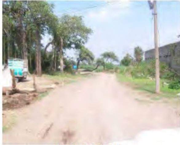
Ch-100m to Ch-200m
