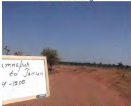
Ch-1200m Junction LHS
