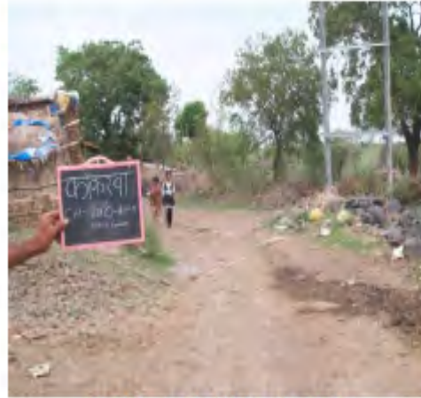
Ch-300m to Ch-400 junction & DP
