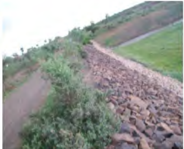
Ch-4000m to Ch-4100m Pond RHS
