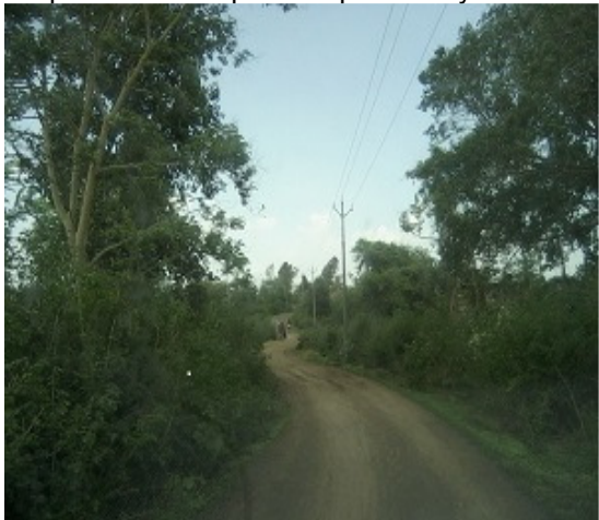
Typical road condition in proposed chainage
