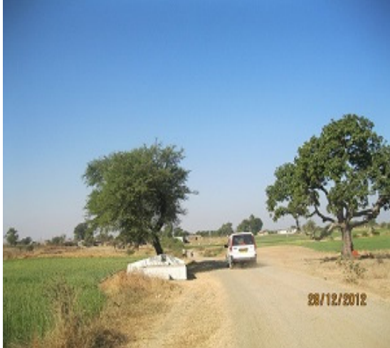
Typical road condition in proposed chainage
