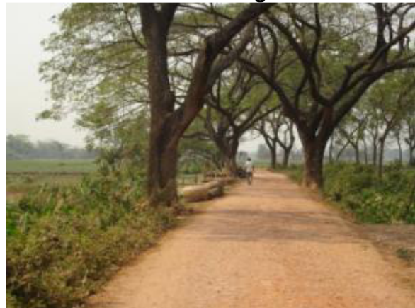
Photo 6: Road in North 24 Pgs -Teghoria Dakshin to Balipur Dakshin considered for upgradation
