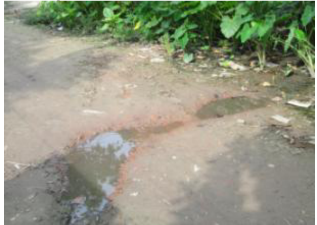
Photo 10: Water stagnation on road Mollapara to Uttar chakla in North 24 Pgs
