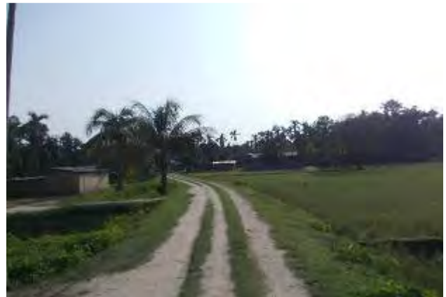
Corridor at 1+900km
