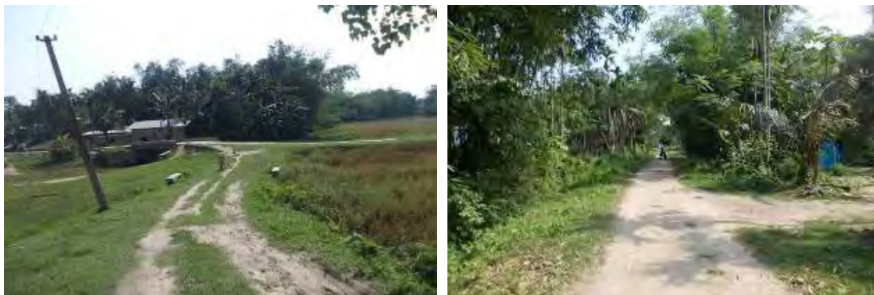
Existing Condition of the Road
