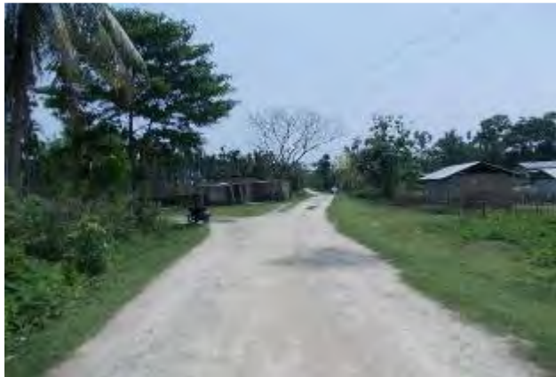
Corridor at 0+200km
