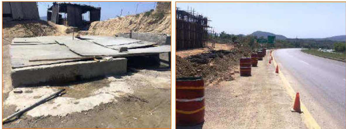
Photo 15 & 16: Water tank of batching plant is protected with wooden sheet. Traffic Management is shown on M1 (Construction Site at RD 0+000). Contractor has installed traffic sign boards at start of work zone on M1. Further traffic signs will be installed as per TMP.
