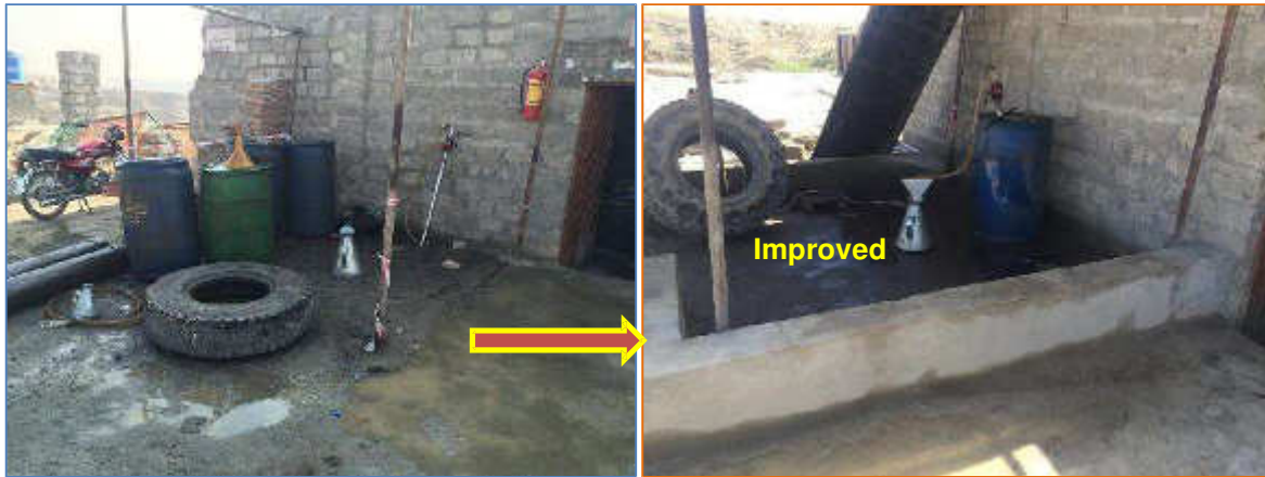
Photo 13 & 14: Fuel Storage Area at Batching Plant site is now improved.
