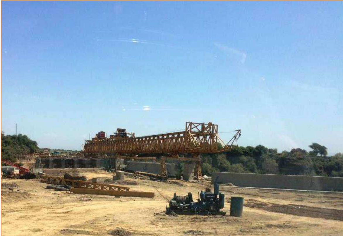
Photo 19: New technology introduced on package 1 for uplifting of girders from casting yard to bridge. This technology is safe and useful in shifting girders.
