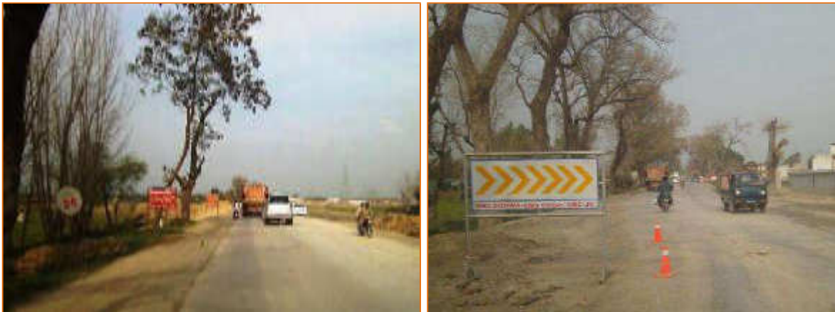
Photo 20 & 21: Traffic Management on Package 1.
