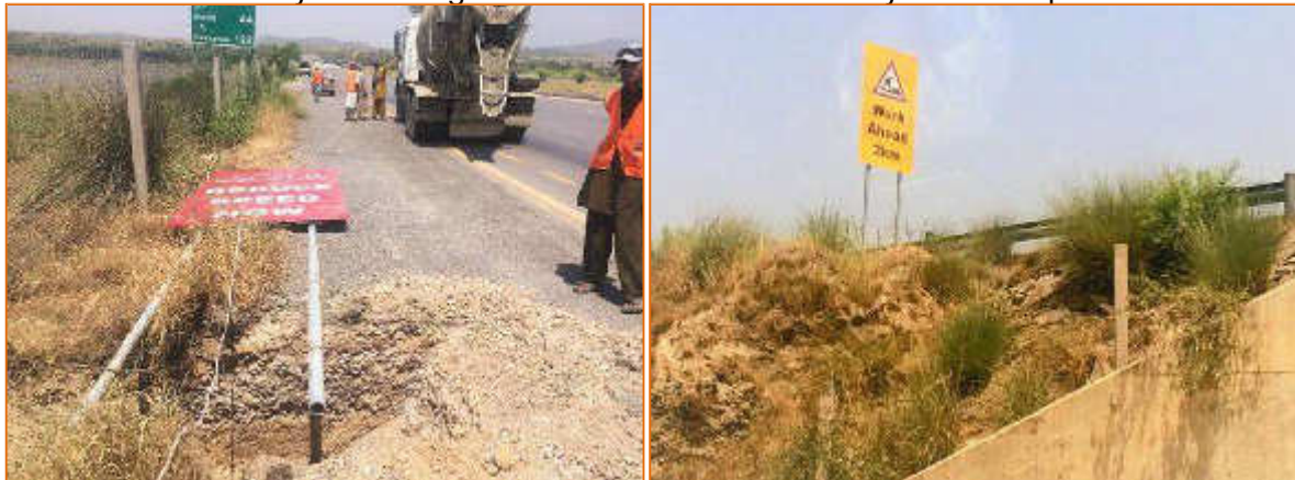
Photo 3 & 4: Traffic management on package 1. Contractor has placed traffic sign boards on M1 for construction work. Traffic Police of Motorways are involved in plan.
