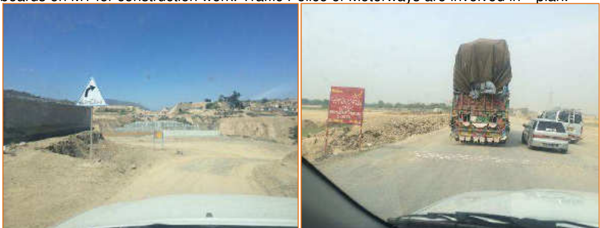
Photo 5 & 6: Contractor has erected different sign boards for guidance and warning of traffic on RoW and on Jarikas road. On Jarikas road speed control measures are taken and work information sign boards are installed.
