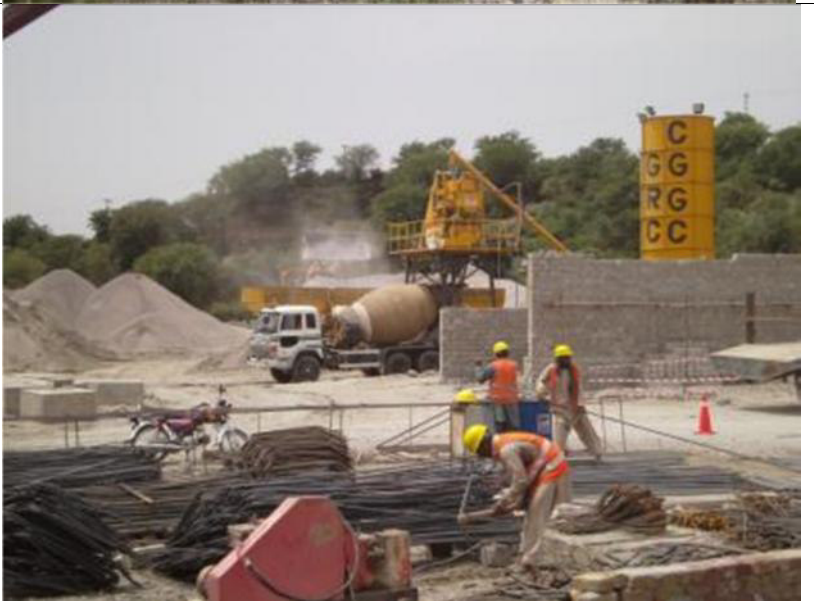
Photo; 9 Batching Plant at 5+260 is operational while steel workers have worn PPEs at Steel Yard Area on Package 1.
