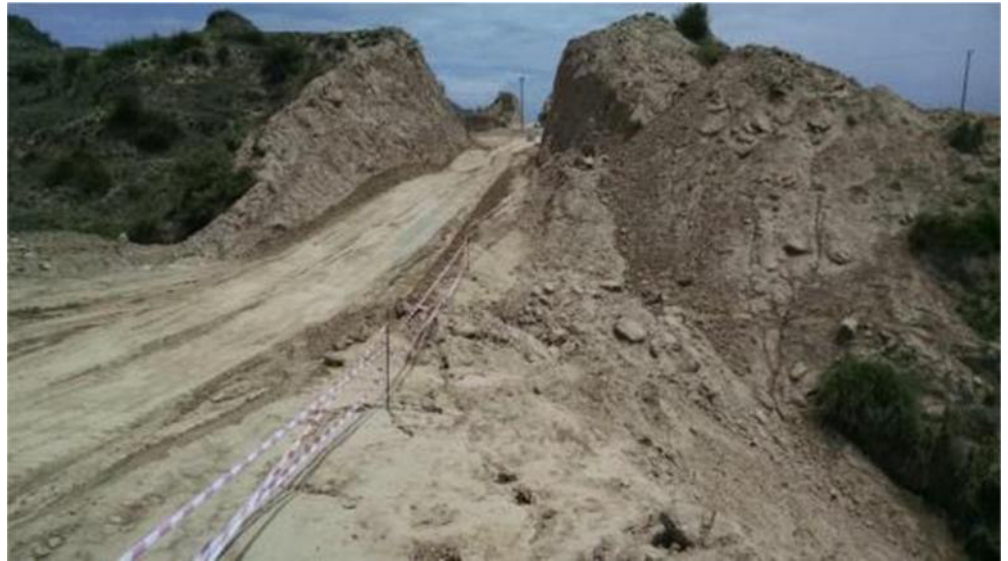
Photo 19; Project ROW access route developed by Contractor on temporary basis.
