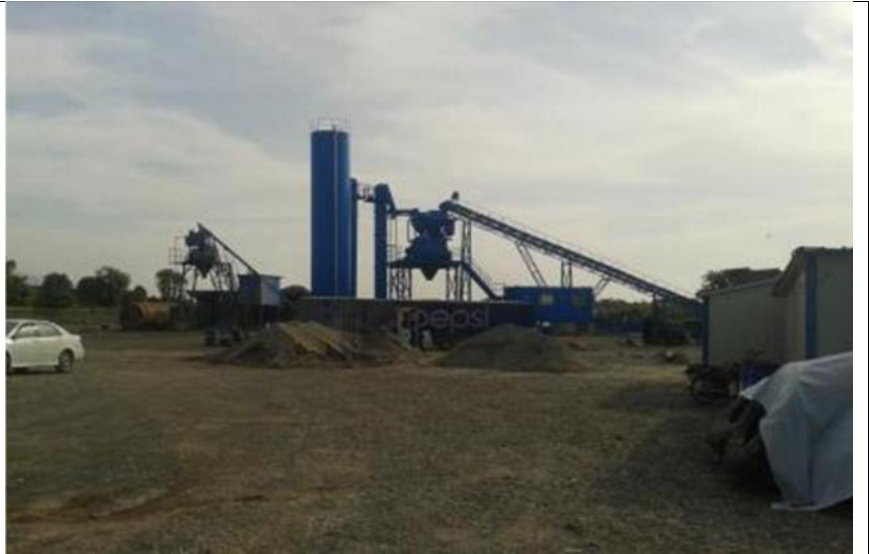
Photo 1; Contractor has installed Concrete batching Plants at RD 28+200 for concrete work of Package 2.
