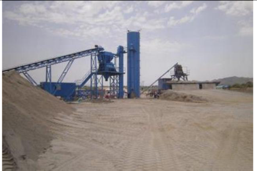
Photo 35; Contractor has installed 2 Concrete batching Plants at RD 28+200 for concrete work of Package 2.
