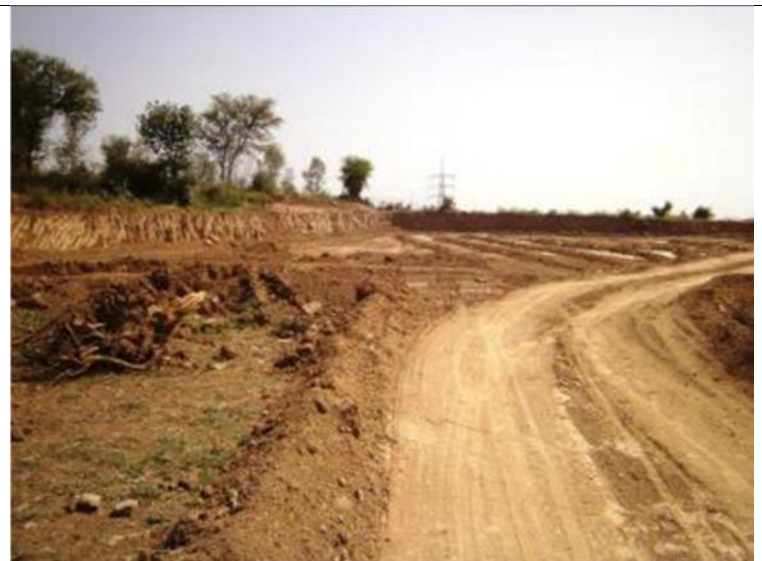
Photo; 34 Borrow area is utilized at RD 31+000, quality test is done on package 2. Contractor has started restoration of this borrow area.
