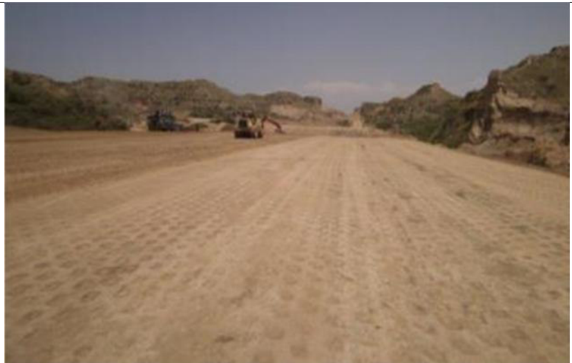
Photo 26; Earth work in progress.
