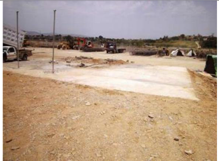
Photo; 33 Fuel Storage areas under construction at Base Camp. Two big Oil Storage Tanks are underground in concreted room and covered from top. Fuel filling dispenser will be placed at this site for filling.
