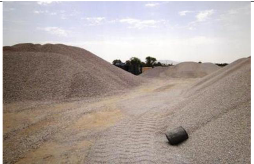
Photo 36; Construction Material Stocked at batching plant site for concrete work. Material
