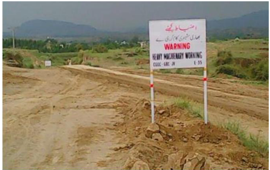
Photo 16; Traffic Warning sign board at Km 1+000 on Package 1. Water is sprinkled by CGGC-GRC.
