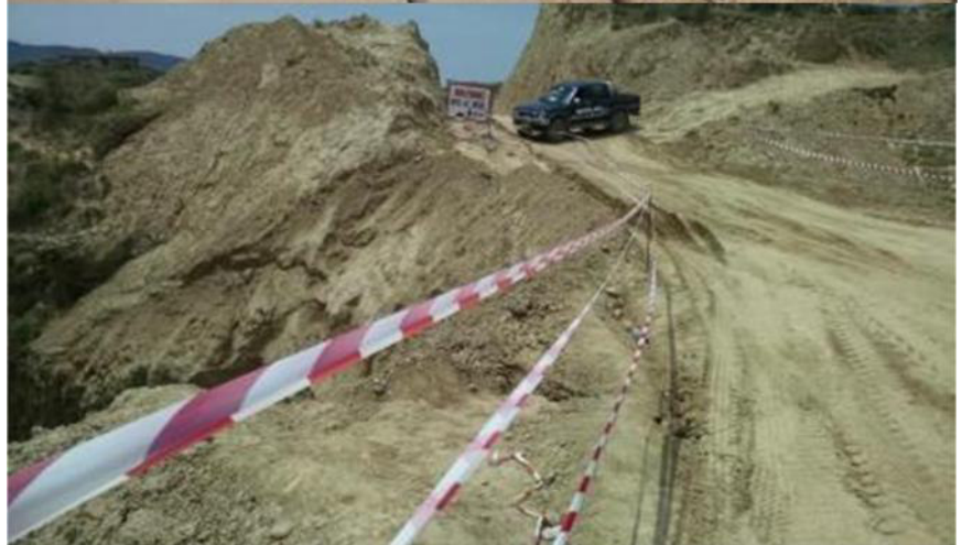
Photo 18: Installation of traffic sign at RD 0+888 with reflecting tap for safety of contractor traffic movement.
