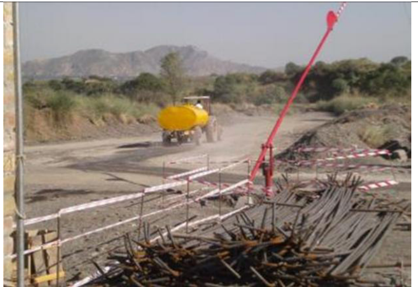
Photo 7: Water Sprinkling on Package 2 for dust suppression in front of base camp.
