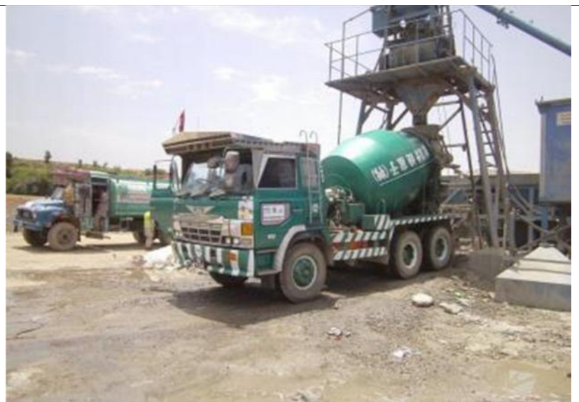
Photo 37: Batching Plant -1 is operational while calibration of plant -2 is done.
