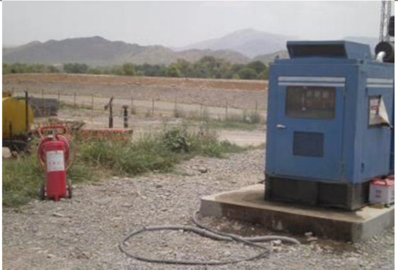
Photo 30; Generator at Main Office site, placed concrete platform with a fire extinguisher. Fire Extinguisher is full and ready for handling fire accident. (Package 2)
