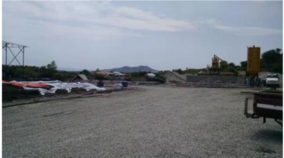
Photo 22: Housekeeping and dust suppression at camp site in May 2015.
