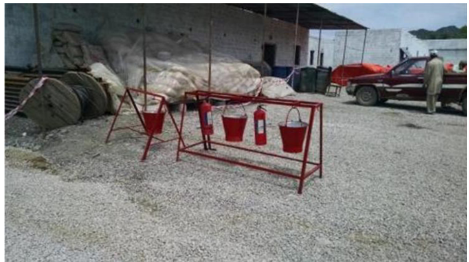
Photo 24: Fire Extinguishers at Camp site of GRC.
