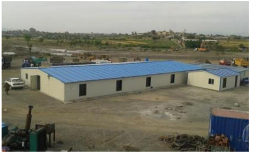
Photo 2; Labour Accommodation at Camp site at RD 28+200.
