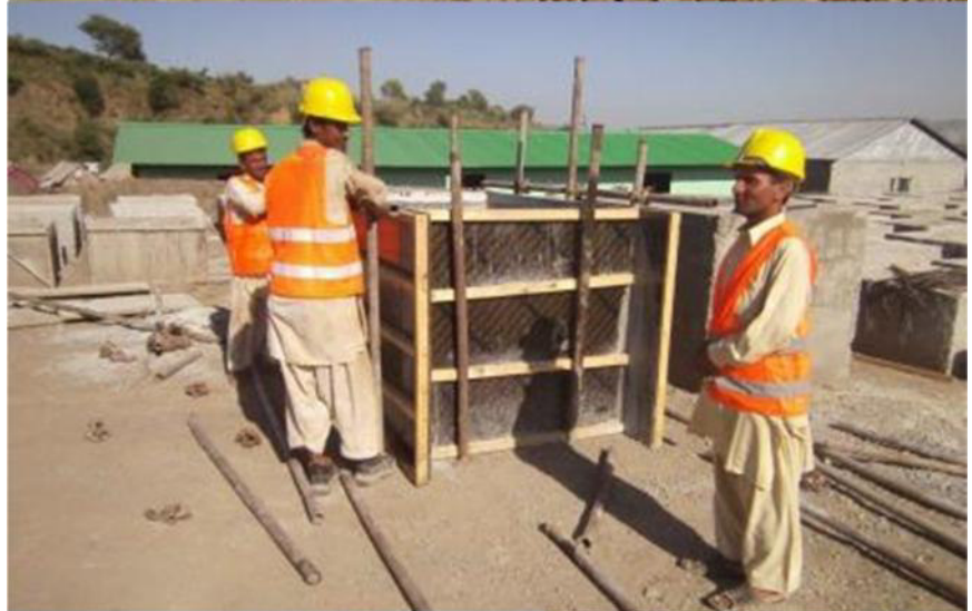
Photo 17; Workers at PC Yard Area (Concrete Blocks) have worn PPEs but few have no Safety Shoes. Contractor is advised for full compliance.
