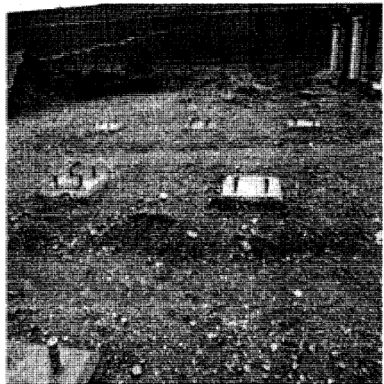
Figure-4: Foundation are completed for line bay at Pishin GS
