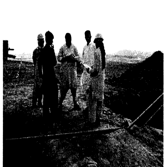
Figure-2: Foundation is being concreted near Pishin at Loralai – Quetta TL
