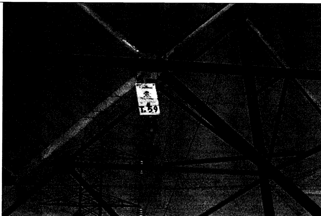
Fig.2 Safety plate and anti climbing device installed at Bagh - Hattian T/Line
