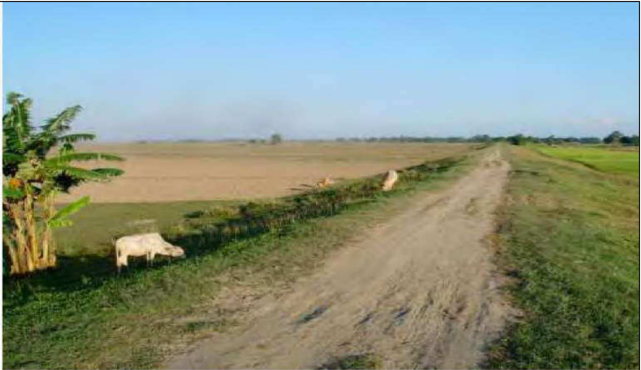
Existing Embankment along the Brahmaputra River
