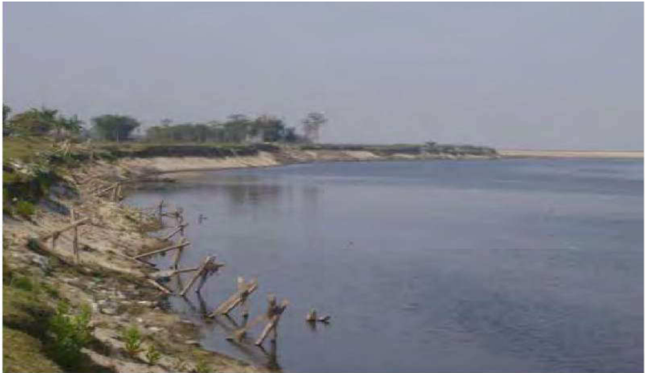
Riverbank Erosion (at Sakopara)
