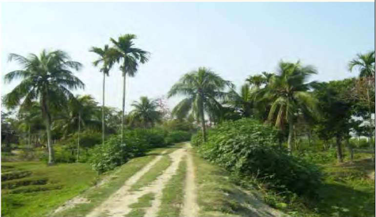
Existing Embankment along Kaziranga National Park Border
