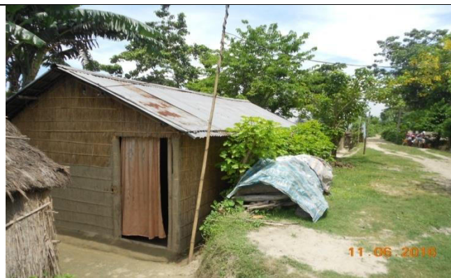
View of Existing palasbari
