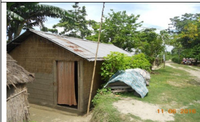
View of Existing palasbari
