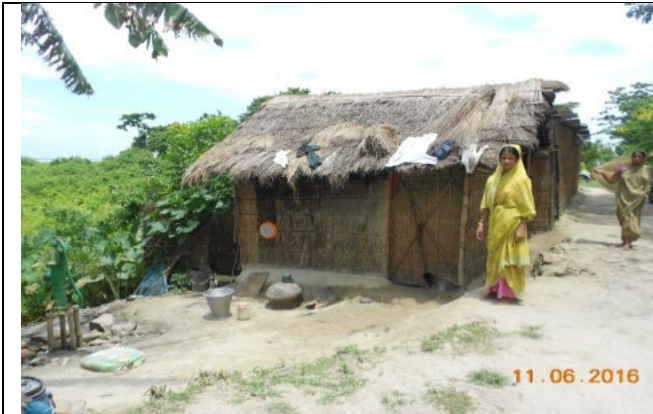
View of the impacted house of Palasbari
