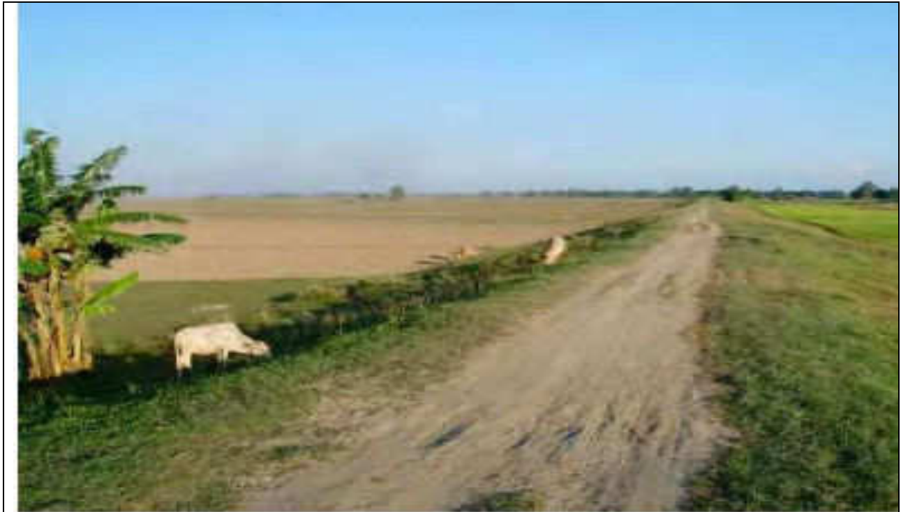
Existing Embankment along the Brahmaputra River
