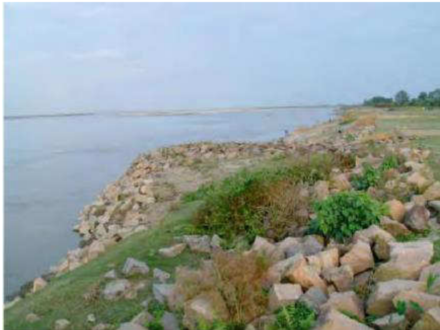
Plate 8: Existing Bolder Flow Deflector (near Gumi)
