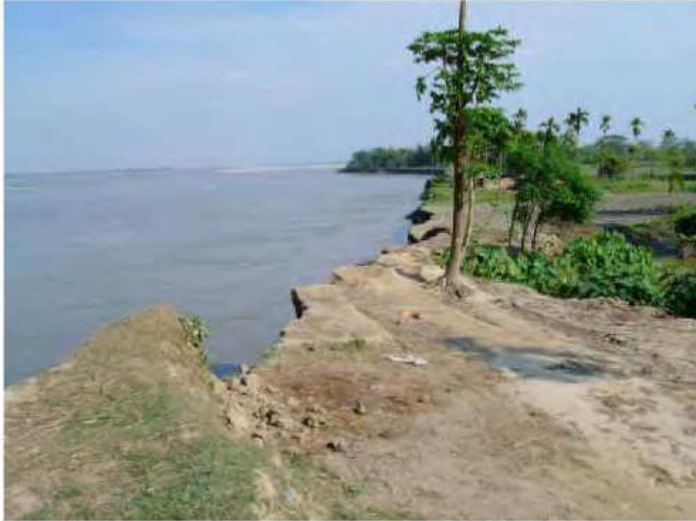
Plate 13: River Erosion near Gumi site
