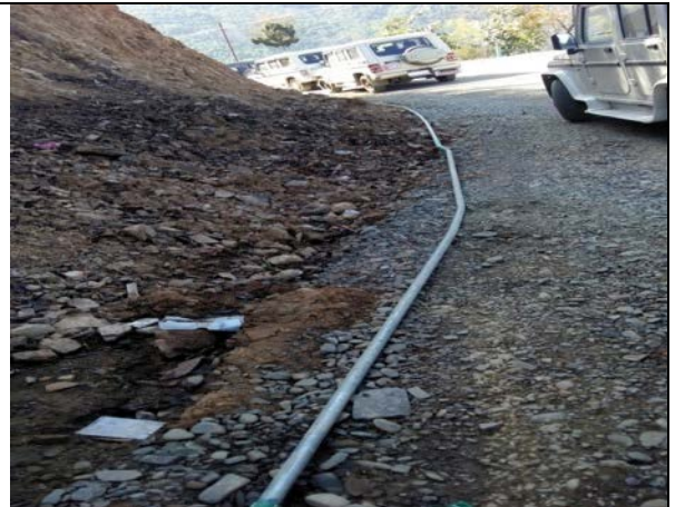
Water supply pipeline laid by Contractor for villages
