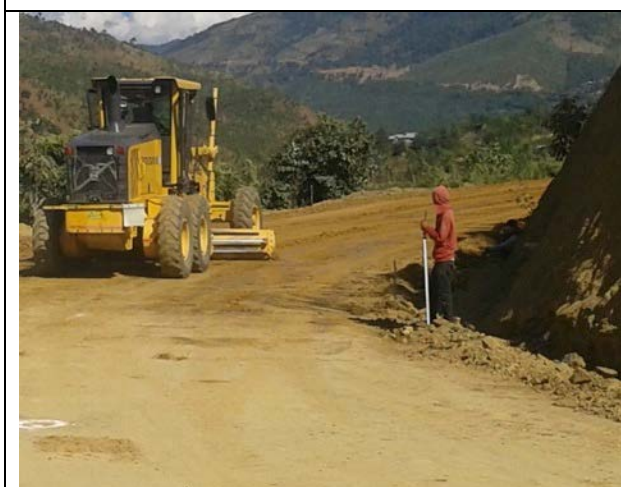
Sub grade in progress at km. 107+300 on 6 Jan 2015
