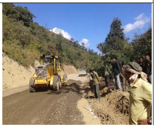
Laying of GSB at km. 109+900 on 12 Jan 2015
