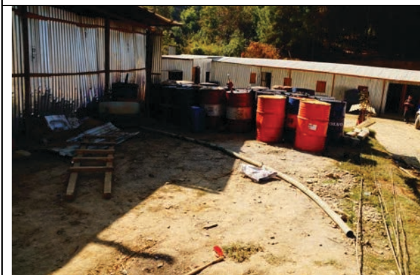
Storage of Lubricant in open area at construction camp (CW2)
