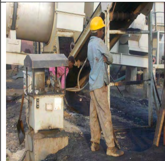
11.Proper use of PPEs required (CW2)
