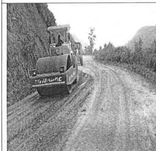
23. Preparation of Sub Grade at Km. 102+10 (CW2)
