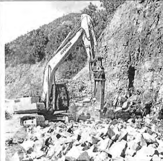
18. Rock Excavation at Km. 105+100 (CW2)
