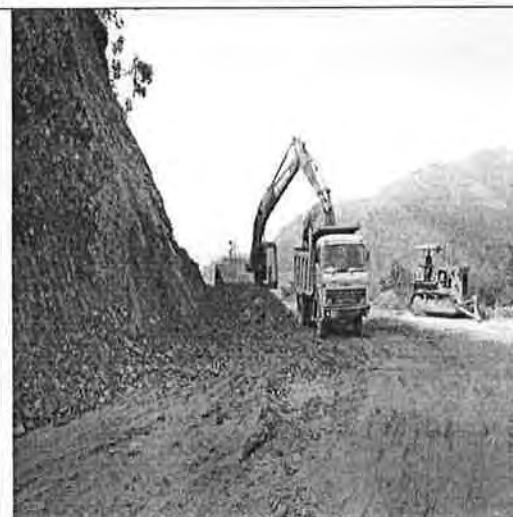
24. Landslide removal at 99+250 (CW2)
