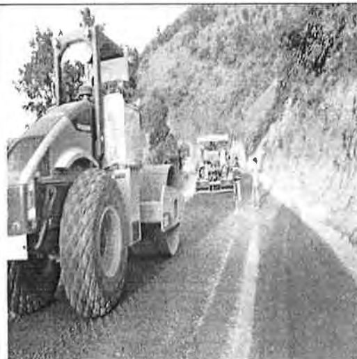
22. Laying of WMM 1 st Layer at 108+150 (CW2)
