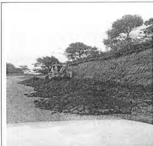
19. Slope correction and surface dressing at 37+100 (CW1)
