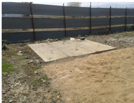
Septic tanks with soakpit at camp site at Mahanadi bridge site in ST-1
