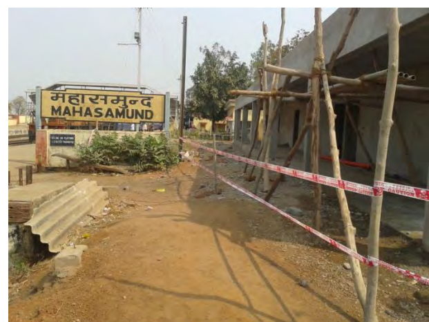
RT-2: Barricadings at site of construction of station building at Mahasamund Railway Station for Public Safety
